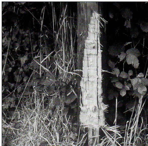
Figure 4. Mowing machine damage.
