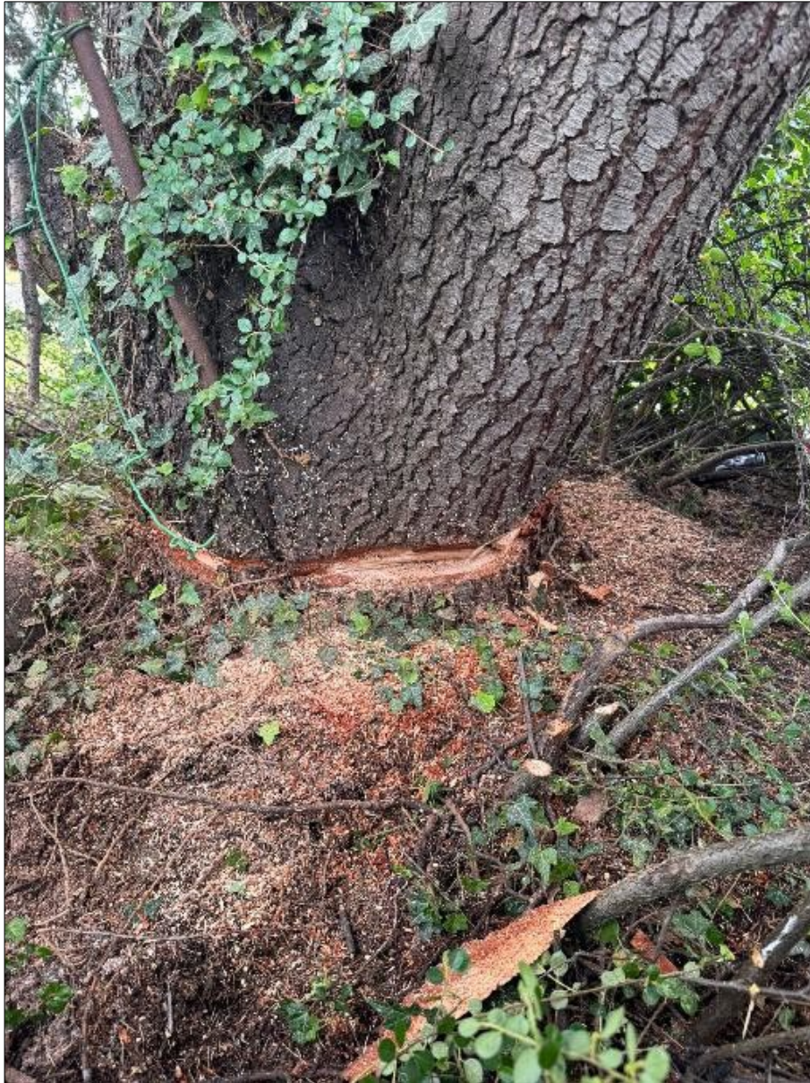
Figure 12 Preparation for Felling
