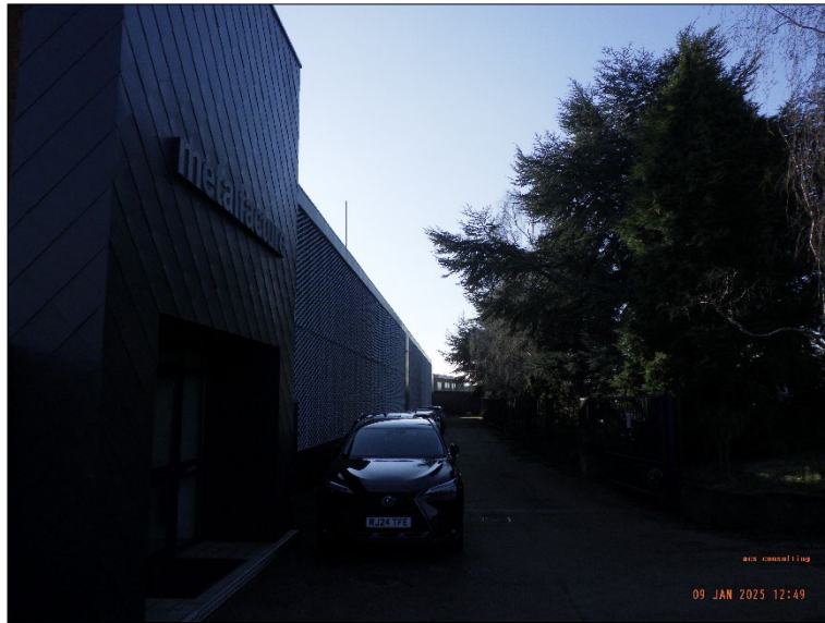
Figure 9 – Poor relationship with offices
