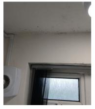
Moderate black mould spores in bathroom.
