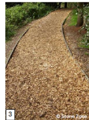
3 Timber edged bark mulch path through existing vegetation. Exact route to be determined on site to minimise impact to existing vegetation.
